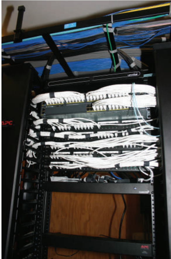
Redundant cabling systems supporting 1,000 video lottery terminals (VLTs) include 30,000 feet of white Category 6A F/UTP (shown here) as well as 30,000 feet of green Category 6A F/UTP cable.
