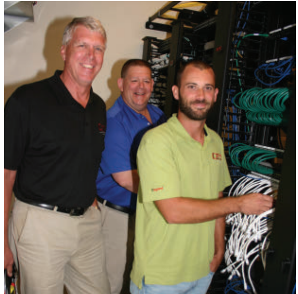
In one of the Racino telecommunications rooms, CRT's Jeff Carr, Dennis Severance, and Lee Olinger make a final check on the installed cabling plant.
