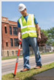
OUTSIDE PLANT Magnetic locator finds buried iron, steel objects
